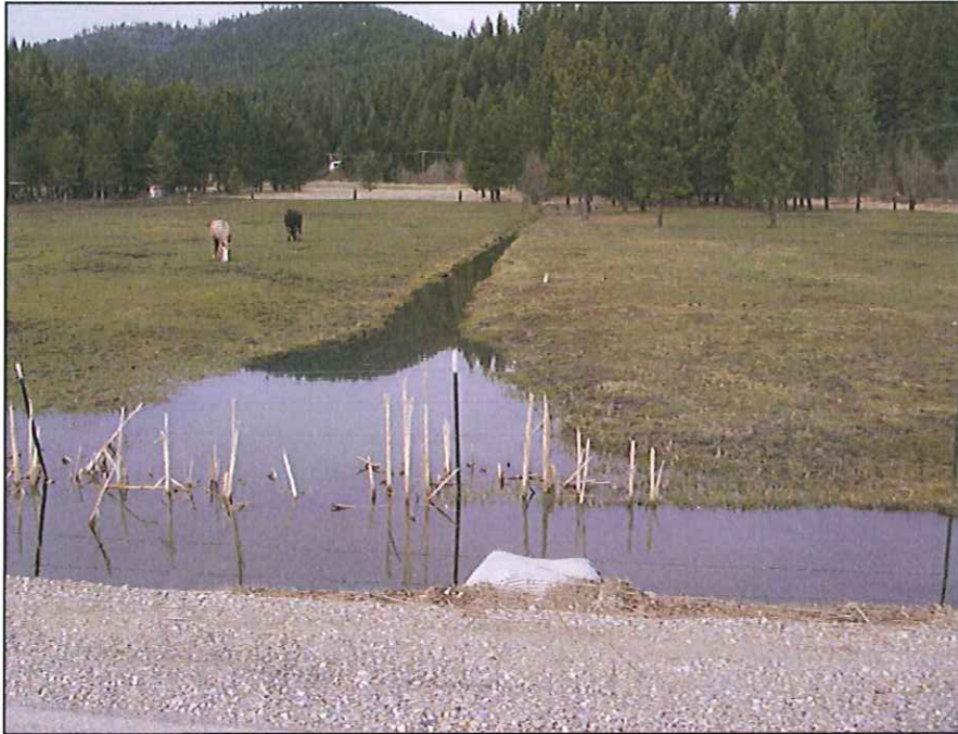
Photo 3: Looking northerly at the Type “F” stream that enters the project area via this 3 foot culvert. This stream travels under West Newman Lake Road and supplies intermittent hydrology into the identified wetlands. Some of the water is impounded by the roadway. Livestock grazing is evident on this adjacent property.
