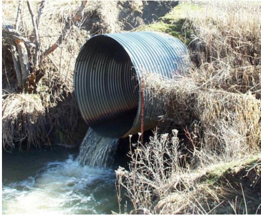
Figure 4. Perched County road culvert
