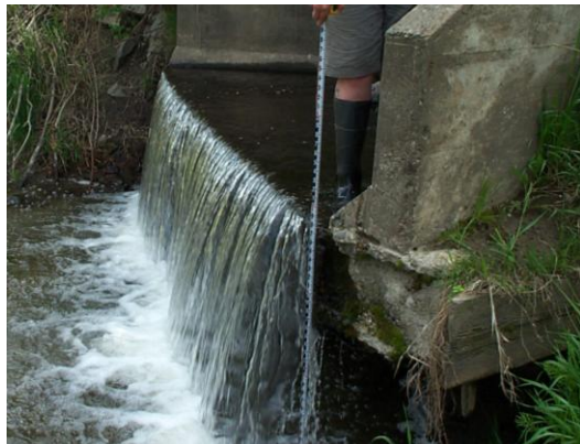
Figure 27. MC-1. US 195 box culvert
