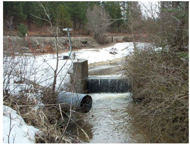
Figure 12. CAC-24, Weir/Dam Structure
