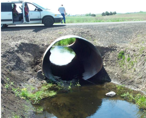
Figure 42. SPC-6. County Road Culvert
