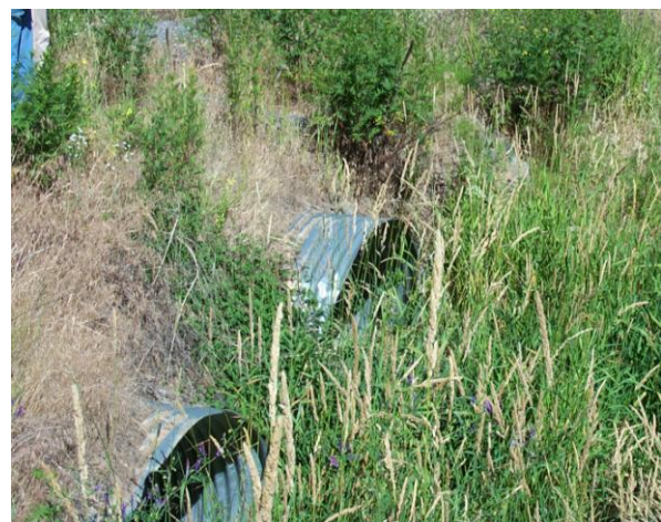
Figure 9. CAC-5, double culvert crossing
