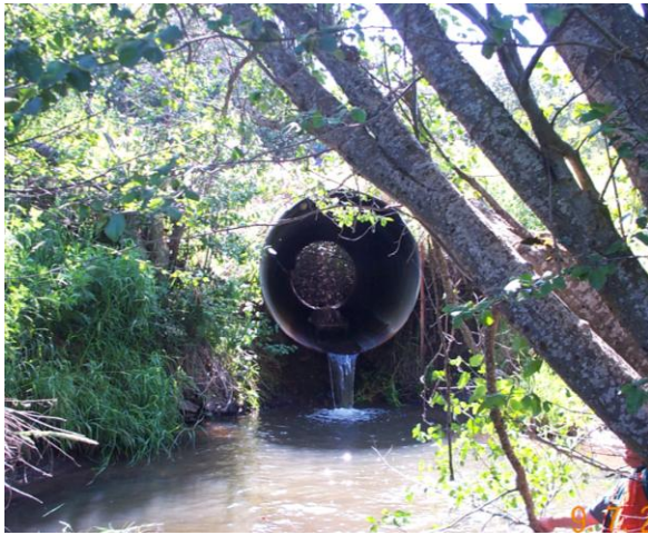
Figure 11. CAC-18, Perched culvert
