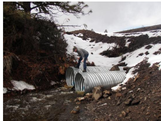
Figure 30. MIN-17 culvert barriers
