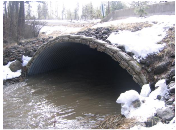
Figure 46. SPC-3, Stentz Rd. crossing
