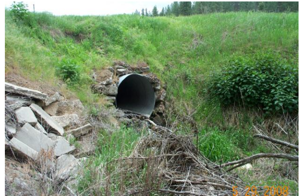
Figure 51. STC-4. Culvert outlet from dam
