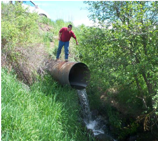
Figure 47. STC-12. Kiesling Rd
