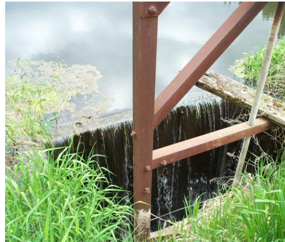
Figure 48. STC-4. Head gate dam
