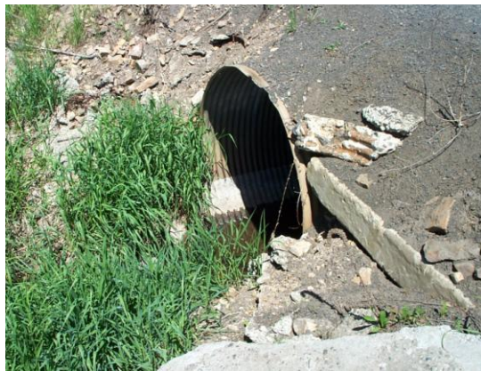
Figure 13. CVC-11. Wheeler Rd. culvert
