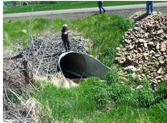
Figure 14. CVC-13. Ham Rd. culvert
