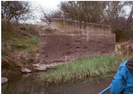
Photograph 4.1. Old bridge abutment.
