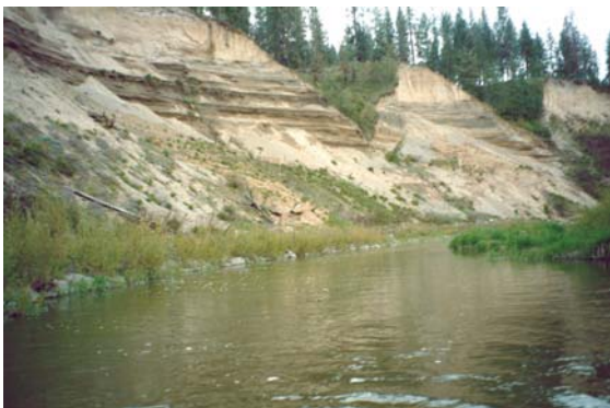
21A.3 Riprap and willows along toe
