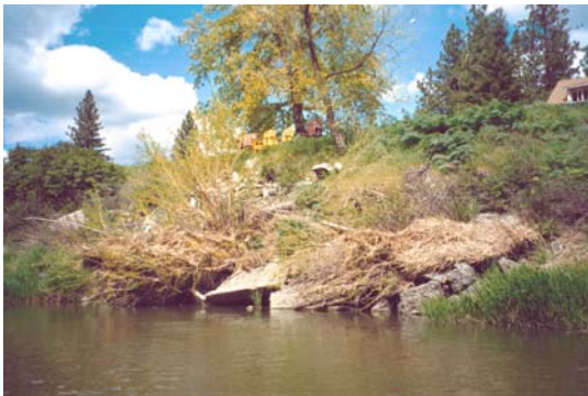
22.1 Riprap and vegetation
