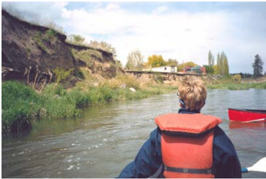
21C.1. Severe erosion (river mile 3.8)
