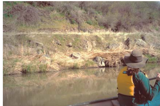
6.2 Riprap along county road
