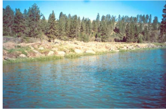
11.2 Riprap serves to stabilize bank and control lateral movement
