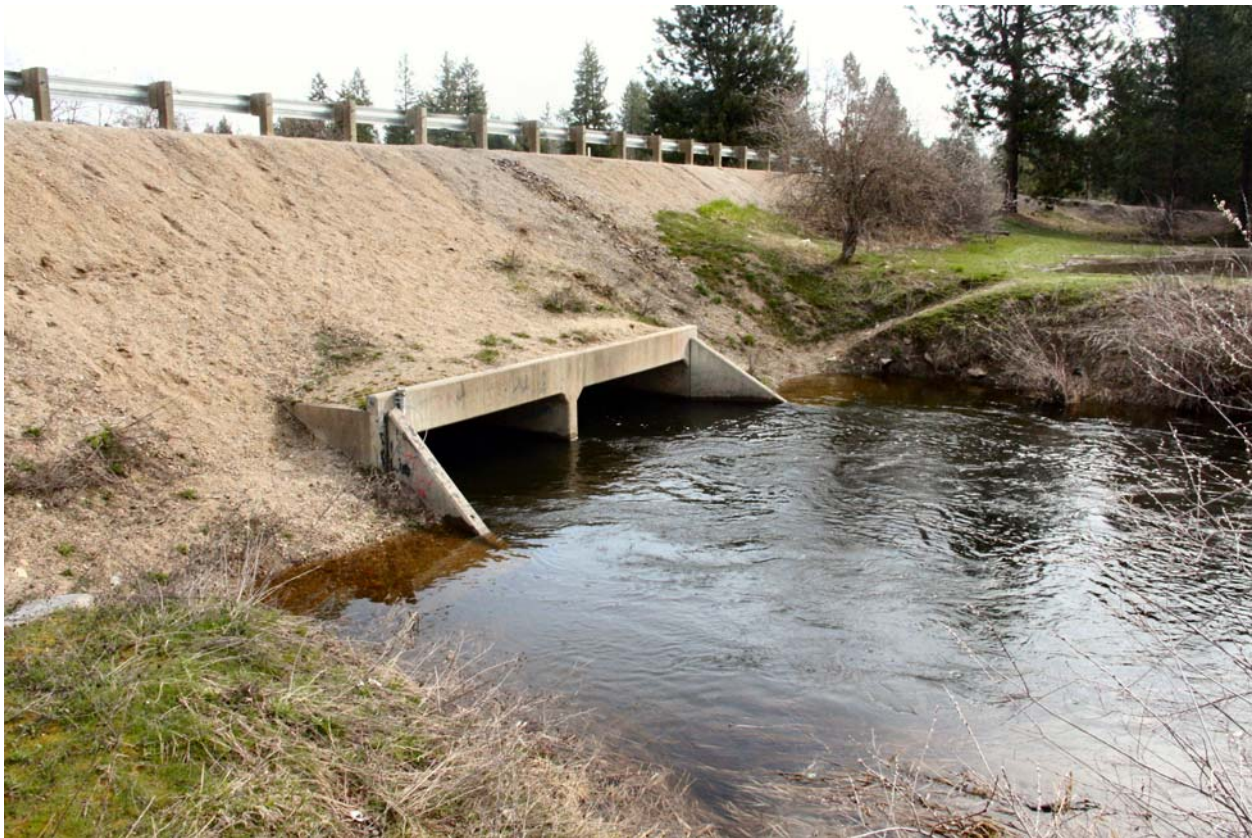
Figure 2-1. Downstream Side of Eloika Lake Road Culverts at Outlet
