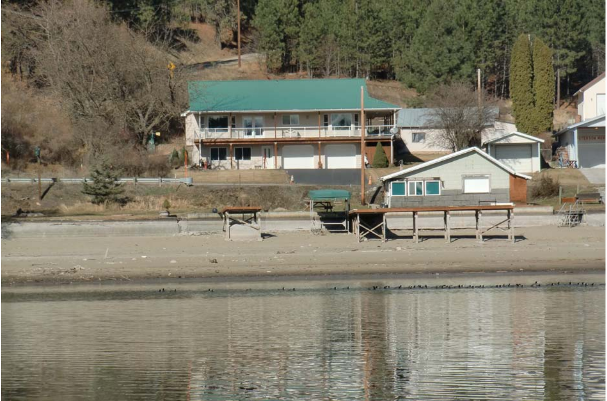
Avista bulkhead removal site in Tum Tum
