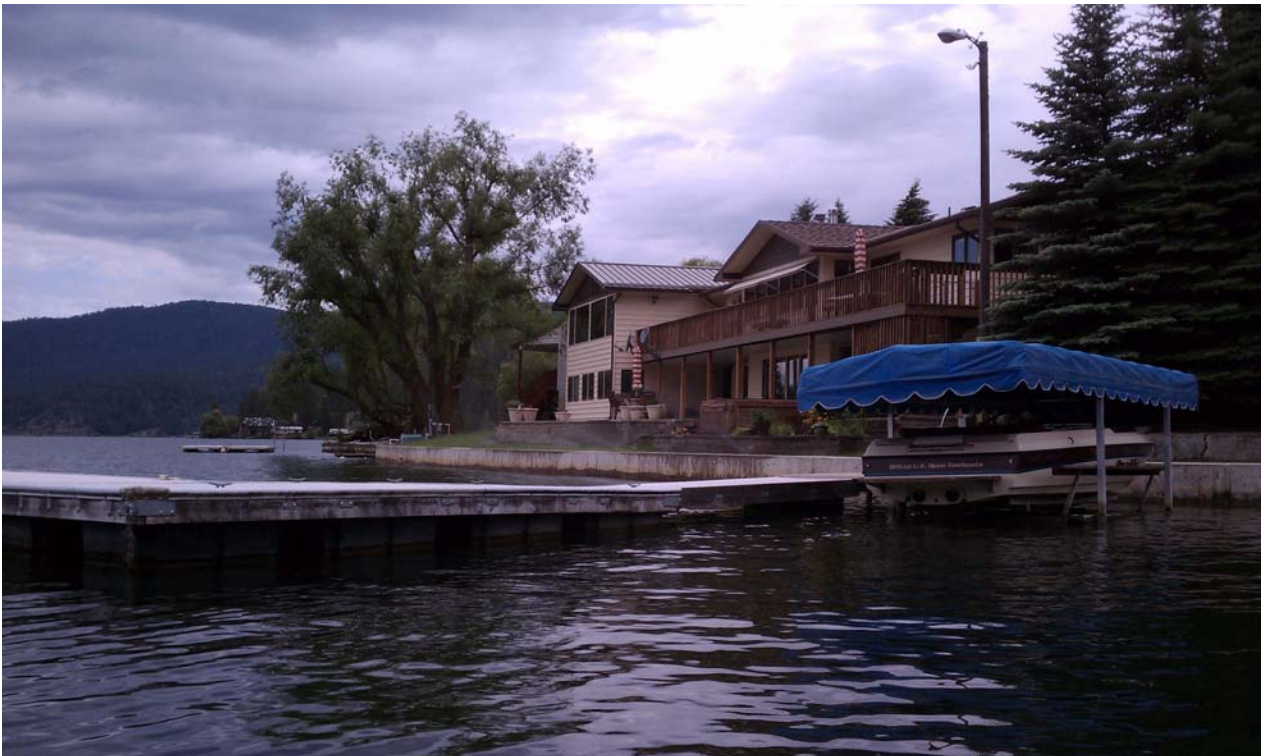
Concrete bulkheads reflect the waves back across the lake
