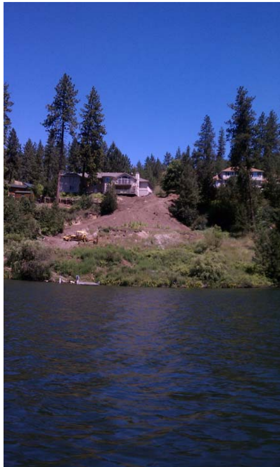
Equipment working above lake, significant exposed soil
