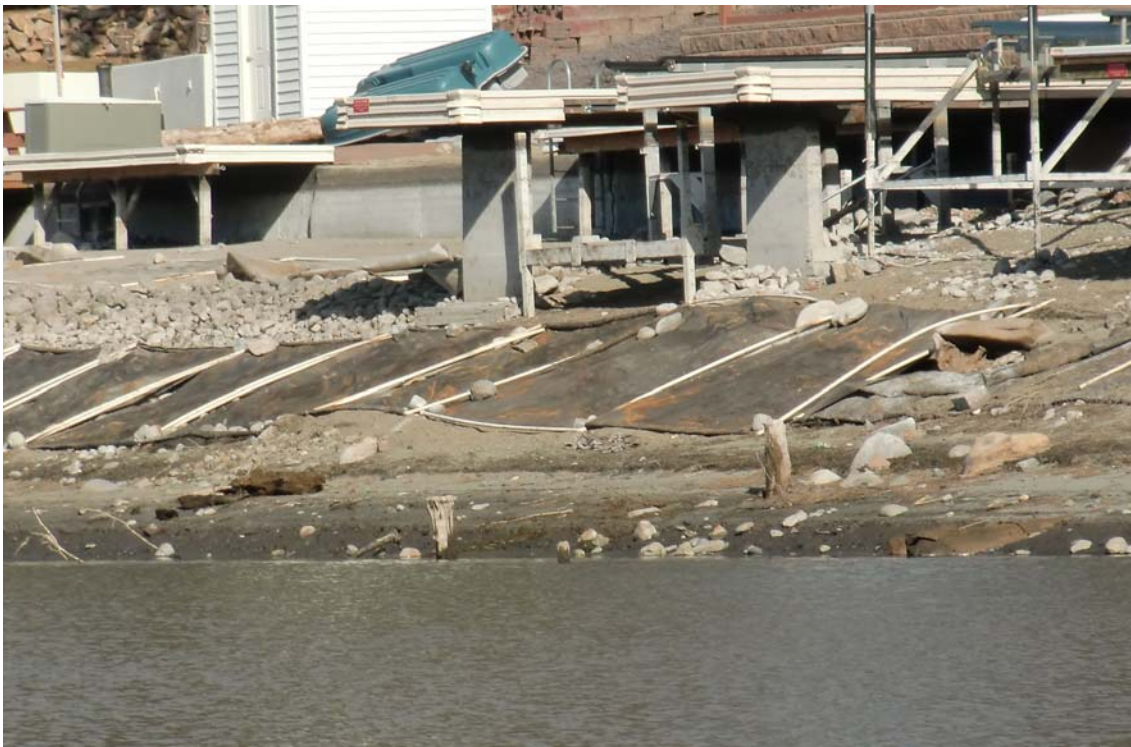
Bottom barriers showing framework and rocks to hold them in place
