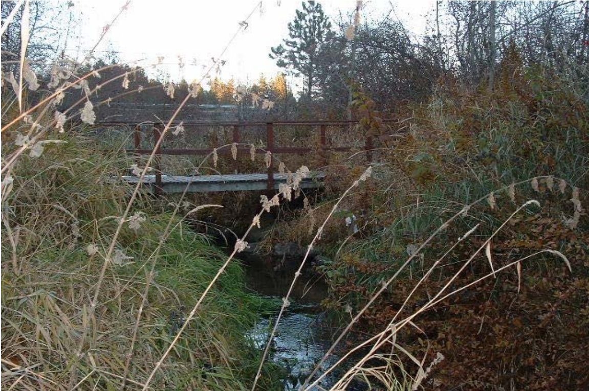
PHOTOGRAPH 55. OTTER CREEK – UPSTREAM VIEW. 10/31/2002, 13:00. Measured Flow: 3.0 cfs. Flow at Dartford: 123-125 cfs. Weather: Overcast, Very Cold. Streamflow Conditions: Stable.
