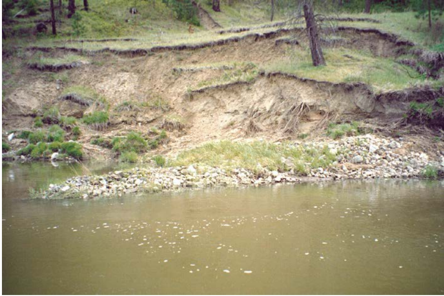
Figure 5. Unstable streambanks in Hangman Valley Floor Area
